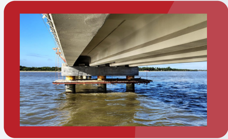
Figura 3. Curing and UHPC protection.
